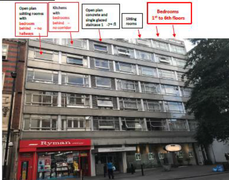
Front elevation 89 GPs W1W 7LX single glazed 1950's concrete construction over 7 floors showing positions of bedrooms and living spaces in flats on 1 st - 6 th Floors - 12 flats single aspect and all single glazed.
