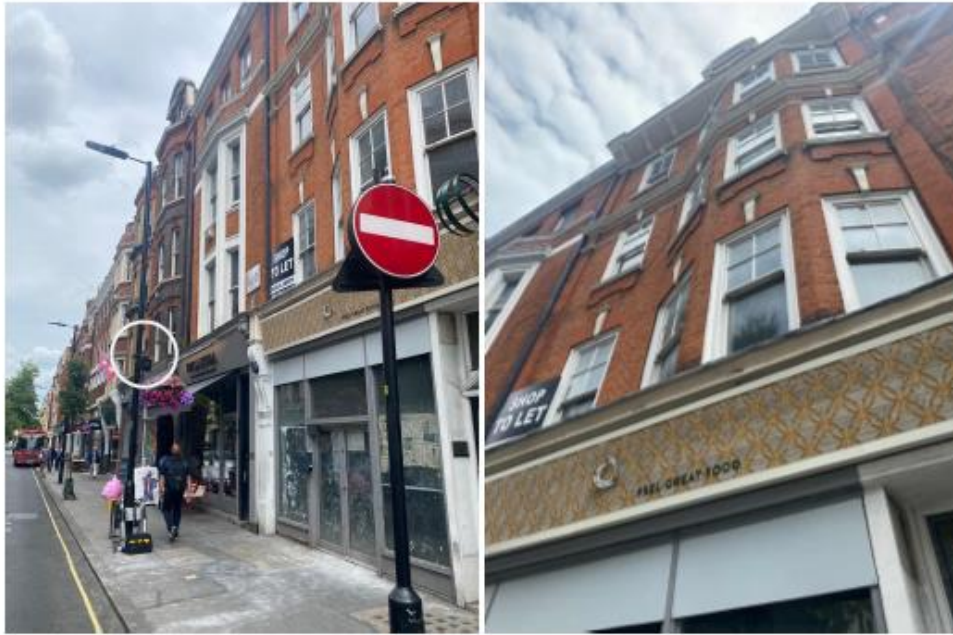
Figure B.1: Noise Survey Photographs
